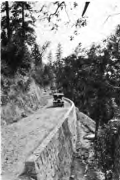
Rock wall protection on Pit River.
